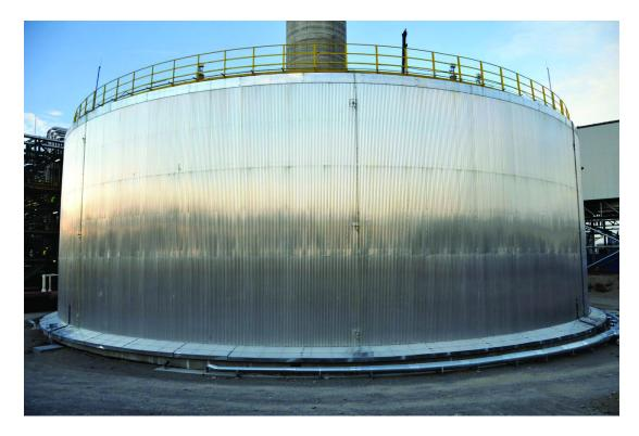
2. Sensible heat storage in action. SolarReserve's Crescent Dunes project in Nevada utilizes sensible heat storage to store up to 10 hours of energy. The molten salt used in the storage process is kept in two large tanks in the center of the solar field. *Courtesy: SolarReserve*
